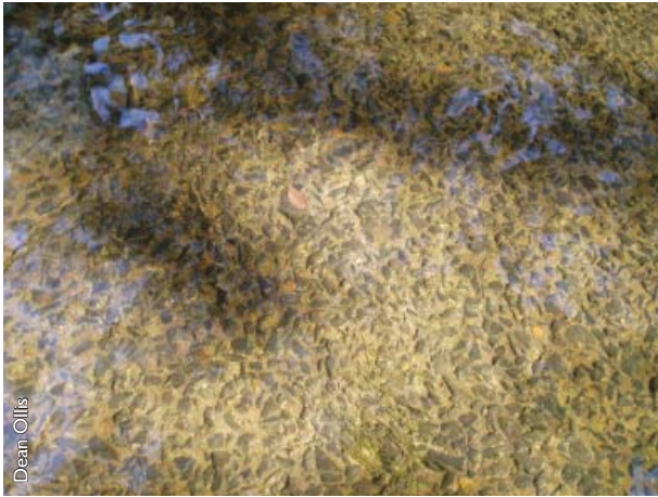
Figure 48. Photograph of the stone and concrete bed of a canalised portion of the Liesbeek River, an example of a substratum type that would fall under the 'other' category.
