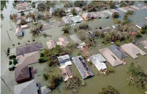
Figura 8.33 KatrinaDestruction.com. New Orleans, LA--Aerial views of damage caused from Hurricane Katrina the day after the hurricane hit August 30, 2005. Photo by Jocelyn Augustino/FEMA
