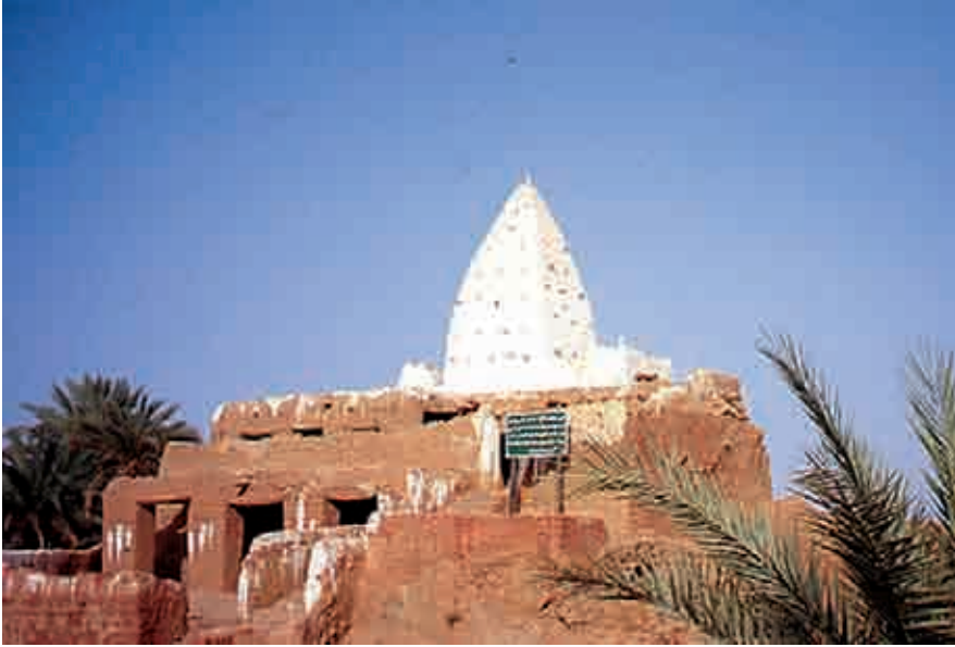
Traditional building, Tamentit Oasis
