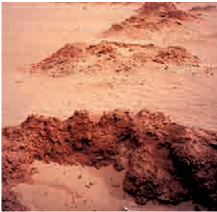
The foggara maintenance shafts are visible on the surface (the conduits are 10-20 m underground). They outline in the desert the trace of the foggaras which may collect water in certain cases from 10-15 km distance from the oasis.
