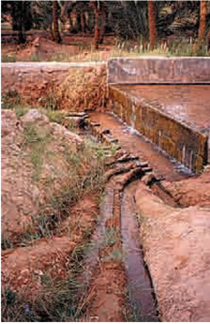
A water distributor, or kasria, at the outlet of a foggara in the oasis
