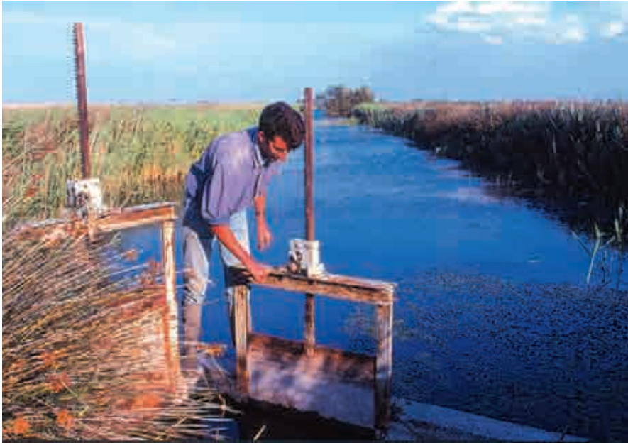
Hydraulic installations, the Camargue
